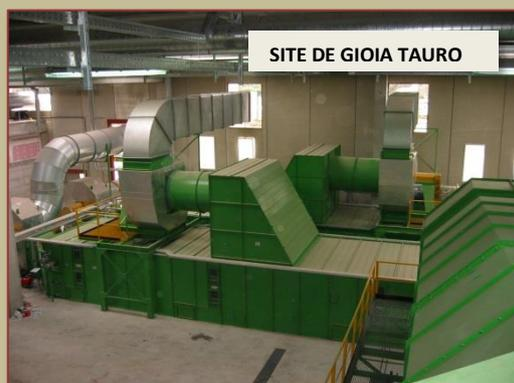
DEUX SECHEURS EXPLOITES EN PARALLELE
